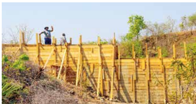
Picture: Construction of sand dam mansinary wall in Neno
